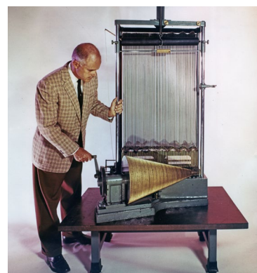
These photographs show Michelson's 80-element analyzer on display ca. 1950-1960. Photos courtesy of the Nimitz Library, United States Naval Academy.
